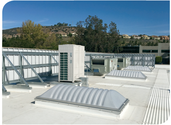
Variable speed compressors used in the Trane® VRF precisely match output to demand levels for comfort and energy savings.
