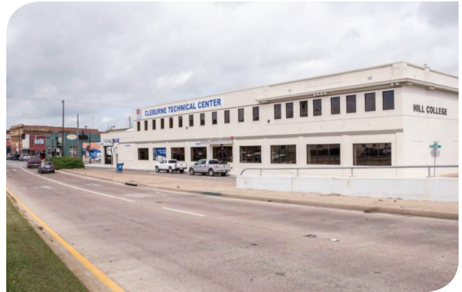
Hill College refurbished an old, historic building for its new HVAC equipment and controls training lab, helping to revitalize the downtown Cleburne area.
