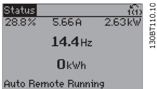
Figure 3.7: Step 1: Turn on the adjustable frequency drive (yellow LED lights)
