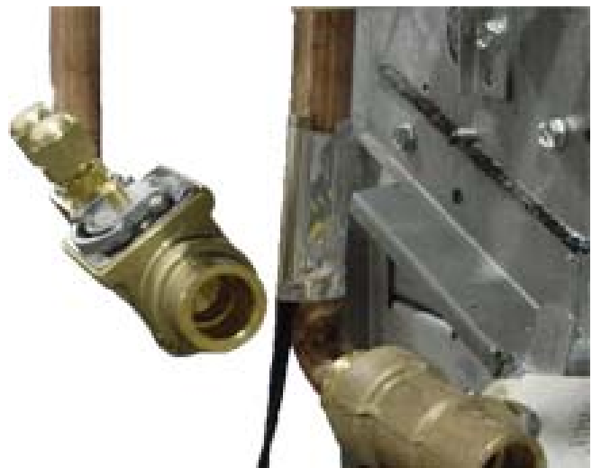
Figure 28. Attach the changeover sensor to the entering water pipe as shown for changeover to work properly
