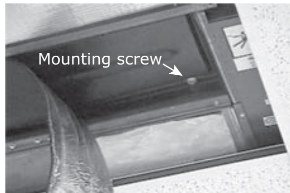
Figure 93. Peel insulation back to see mounting screw
