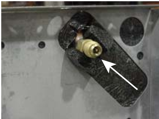
Figure 31. Manual coil air vent with Shrader fitting
