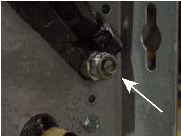
Figure 31. Manual coil air vent with Shrader fitting
