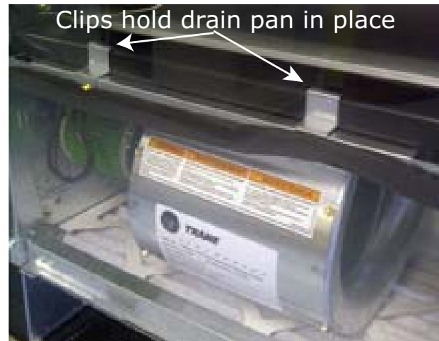
Figure 94. Clips hold drain pan to the fan board
