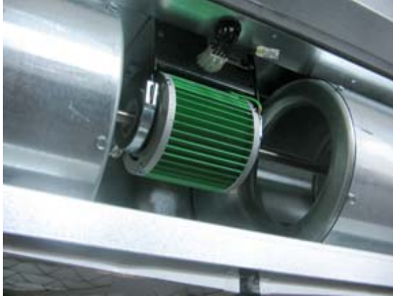
Figure 100. Motor attachment screws are behind motor
