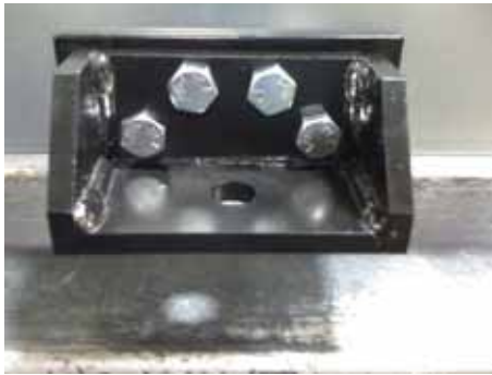
Figure 82. Seismic anchor
