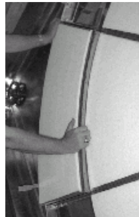
Figure 152. Install outer segment by starting lower end in position and pressing straight in
