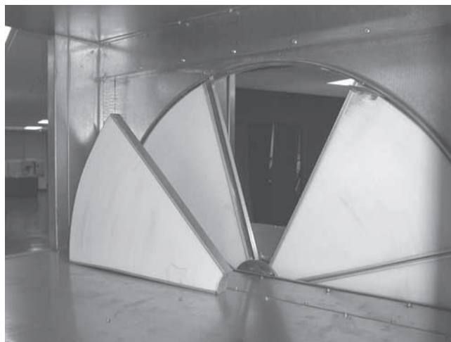
Figure 147. Pull the segment up and out of the wheel frame to remove
