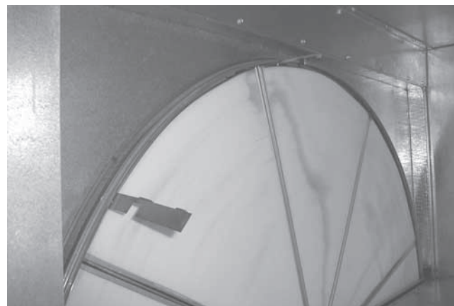
Figure 147. Pull the segment up and out of the wheel frame to remove
