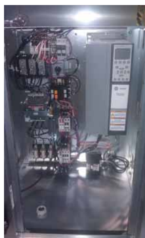
Figure 125. Internally mounted VFD
