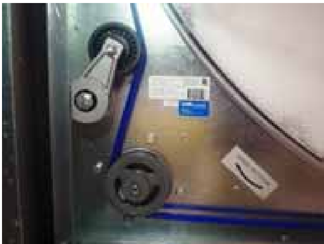
Figure 145. Confirm proper belt tracking on the wheel rim
