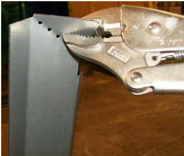
Figure 48. Bend end tabs and apply Butyl tape to flashing.
