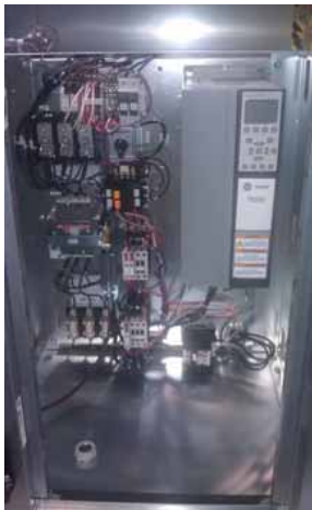
Figure 121. Internally mounted VFD
