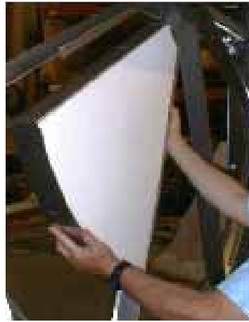
Figure 148. Install outer segment by starting lower end in position and pressing straight in
