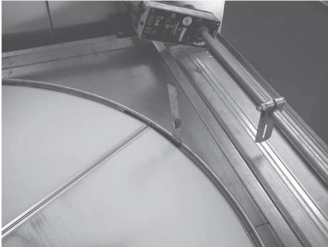
Figure 141. Confirm proper belt tracking on the wheel rim
