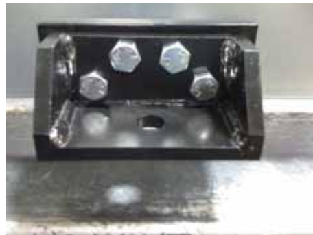
Figure 78. Seismic anchor
