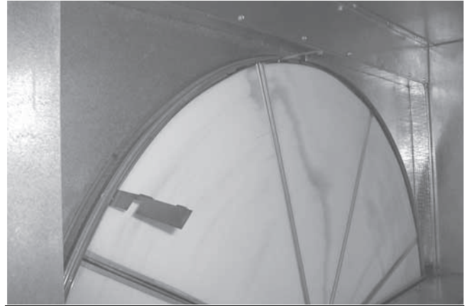
Figure 143. Pull the segment up and out of the wheel frame to remove
