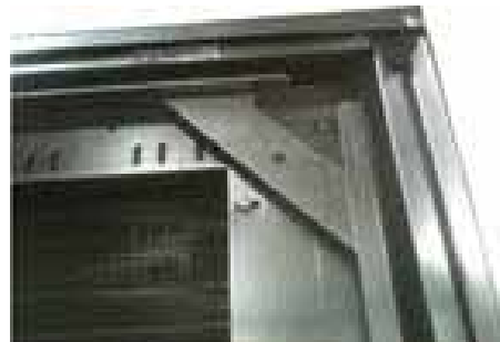
Figure 24. Coil structural gusset
