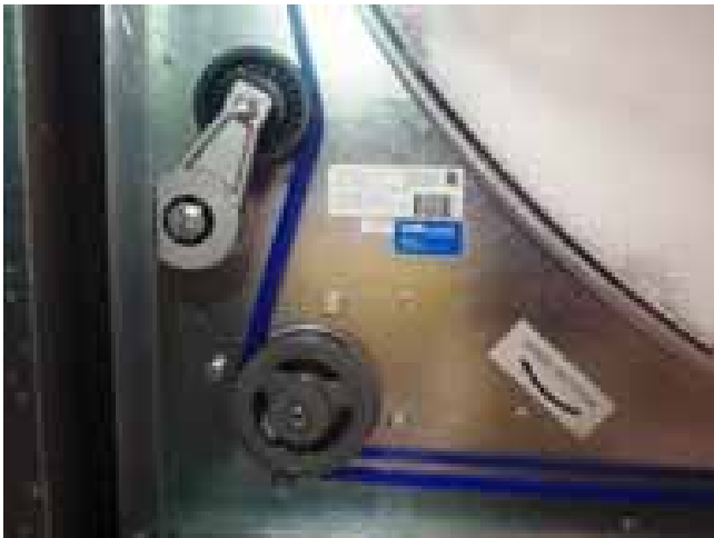
Figure 141. Confirm proper belt tracking on the wheel rim
