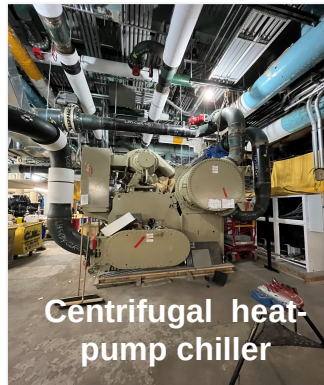
modular heat-pump chillers
