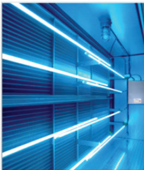
Figure 13. UV-C installation in an air handler
