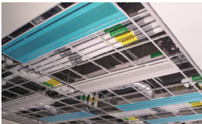
Figure 20. Installed chilled beam example
