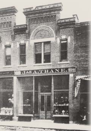
Trane Storefront La Crosse, Wisconsin 1891
