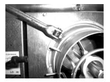
Remove air valve from existing VAV unit by breaking the seal around air inlet and the VAV unit. Once it is loose, remove air valve (see Figure 5, p. 13).
