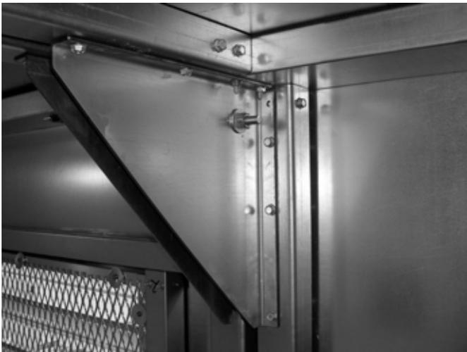
Figure 29. Join internal shipping split frame- Graphic 2
