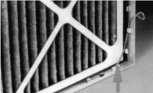
Figure 46. Bag filter show with C-70 fastener
