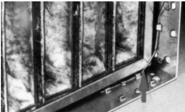
Figure 45. C-86 fastener (shown) or C-77 fastener holds 4-inch pleated filters
