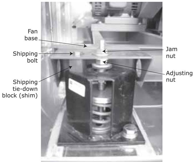
Isolators are selected for distribution of equipment weight, but may not all compress the same. This procedure assumes the base surface is level. Isolators are not intended to be leveling devices.
