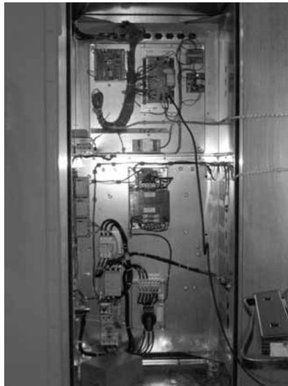
Figure 69. Variable-frequency drive (VFD)
