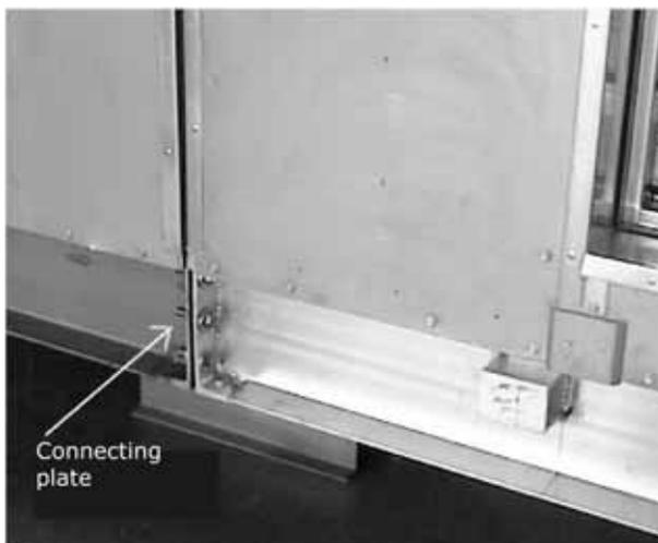
9. Pulling sections together on a flat surface can be done by using chain come-alongs hooked onto the welded square tubes located on each side of the shipping split. These square tubes are designed to fully support the stress of pulling sections together. Sections should be pulled together until mating gaskets make contact and factory-supplied bolts can be installed in connecting plate.
