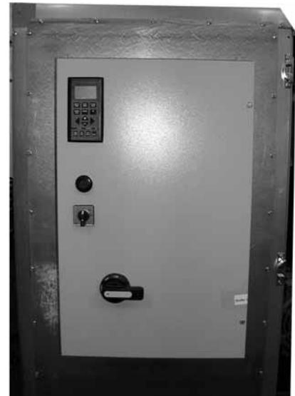
All units with starters or variable-frequency drives (VFDs) that have direct-digital controllers (DDCs) are provided with line voltage to 120 Vac power transformers (see [Figure 67](#)) with power 120 Vac to 24 Vac control transformers (see [Figure 68](#)). [Figure 69](#) shows a typical VFD power box.
