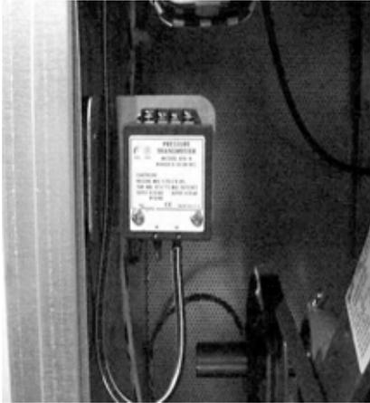
A fan inlet airflow measuring system with a piezometer ring is available on many centrifugal and plenum fans. Each system comes with a differential pressure transmitter. The piezometer ring is connected to the LO port of the transmitter and the reference pressure point is connected to (or actually is) the HI port of the transmitter. See [Figure 77](#).
