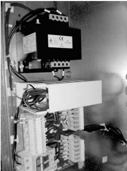
Figure 68. 120 to 24 Vac Control Transformer
