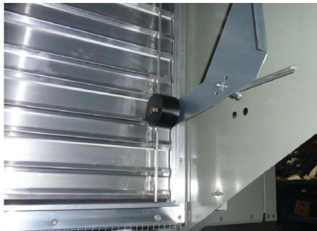
Figure 52. Exhaust damper linkage arm
