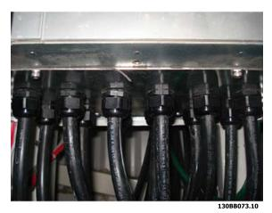
Illustration 3. 35: Example of proper installation of the gland plate.
