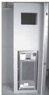
Figure 15. Install chassis centered
