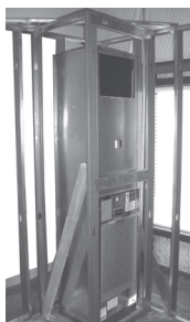
Figure 8. Mock-up of stud placement
