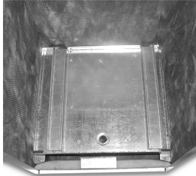
Figure 1. Auxiliary drain pan
