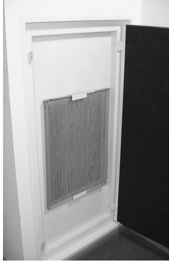
Figure 2. Return-air flush mounted hinged door
