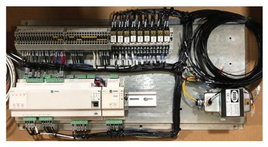
4. Install the new back plate to the main electrical panel with provided sheet metal screws. On 80 to 120 ton units, install timers 7U5 and 7U6 in top left corner of back plate. Connect wires 58C to 7U5-1, 100B to 7U5-2, 36AW to 7U5-3, 71C to 7U6-1, 101B to 7U6-2, and 36AV to 7U6-3. Reference CST Supplied wiring diagram (lines 81 to 88).
