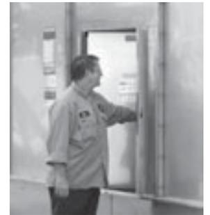
the access doors are 48" high. Small access doors are prohibitive and discourage maintenance, which in turn can impact your operation. Specifying the size of the door will cause some bidders to take exception, alerting you to a potential maintenance headache. Two doors are standard on all Series Quiet Class towers—one in each endwall.
