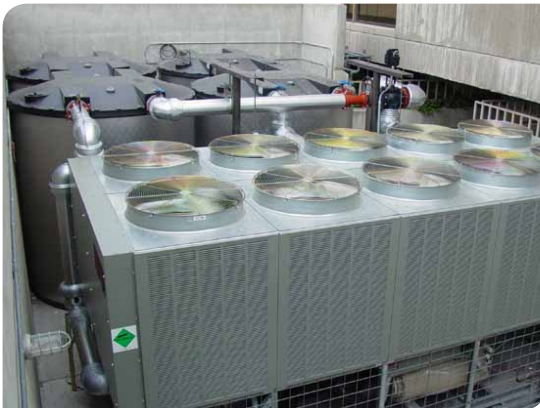
One way Trane reduces energy costs is with a thermal storage system design that uses ice made at night, when energy demand and cost are lowest, to cool the building during the day.
