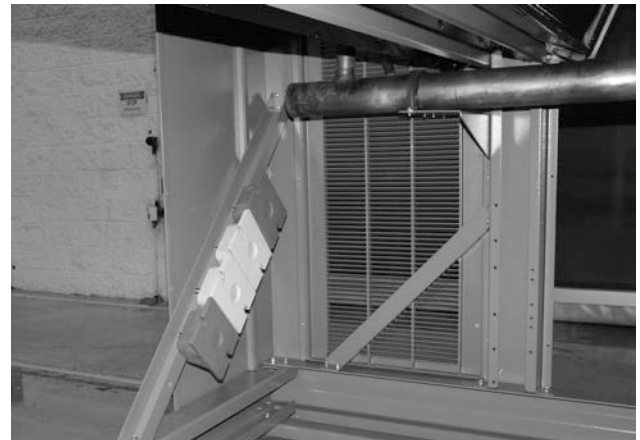
Figure 2. Elastomeric isolators attached for shipping
