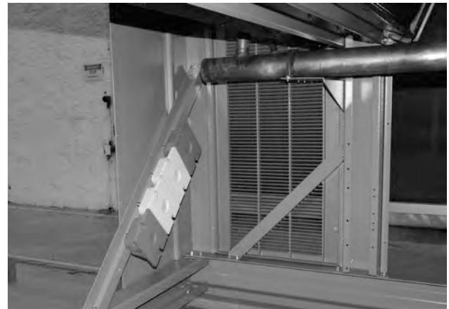
Figure 2. Elastomeric isolators attached for shipping
