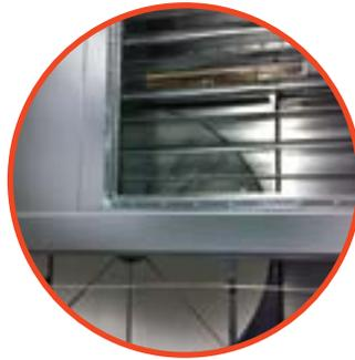
**The patented Trane Dual Exhaust Energy Recover (DEER) system** captures energy that would otherwise be lost by directing exhaust air from a building and its restrooms into a specifically designed energy wheel arrangement that recovers energy from multiple air streams while minimizing recirculation of toilet exhaust — in a single unit with a more efficient fan and motor arrangement.
