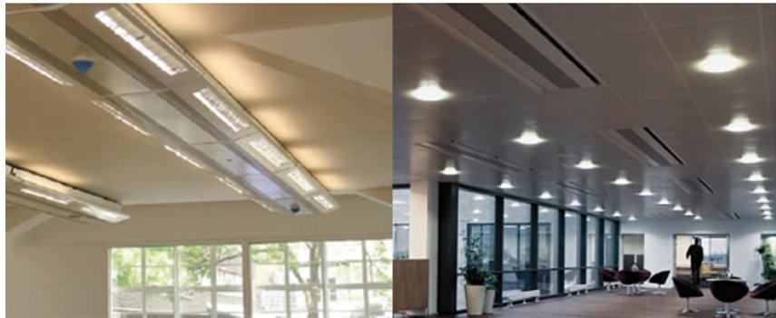
Returning to the same example, four 6-ft long active chilled beams are needed to offset the space sensible cooling load for this 1000 ft<sup>2</sup> office space (Figure 11). Notice how much ceiling area is covered with the beams.
