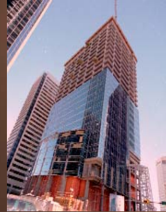
Headquarters building (under construction) Calgary, Canada
