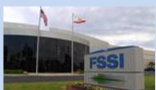
Upgrades at FSSI's 168,000 square-foot corporate headquarters are expected to save $72,000 per year.
