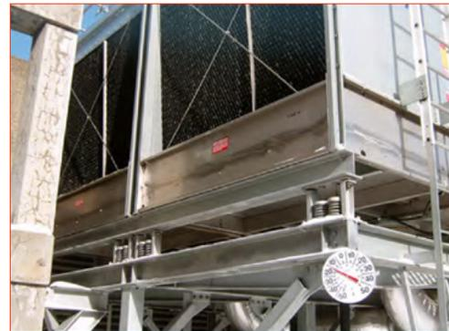
Cooling tower operating during freezing conditions
