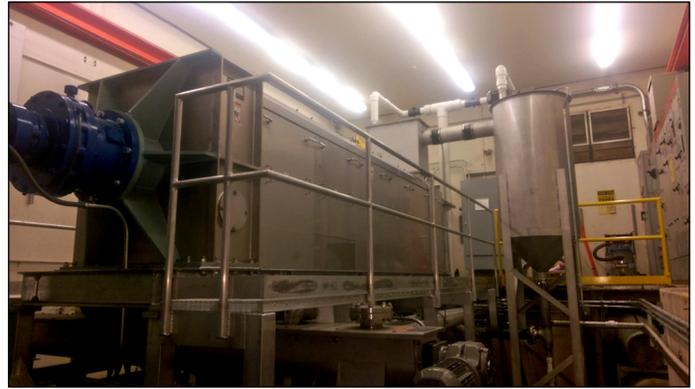
*A single dewatering screw press replaced two aging centrifuges, helping to improve reliability and reduce energy consumption.*
