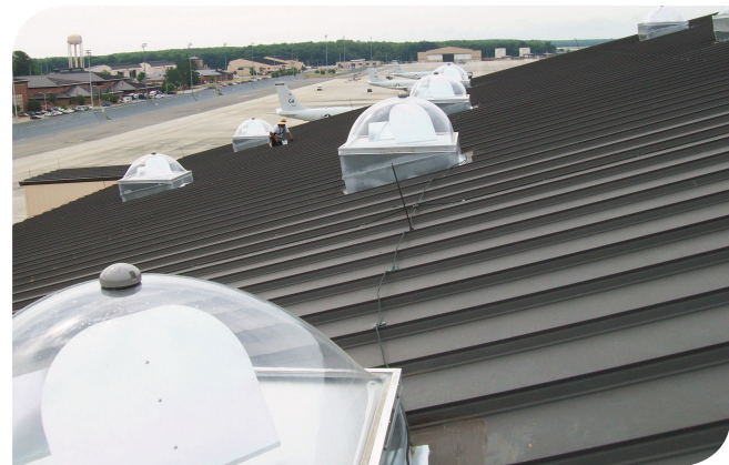
Over 300 skylights installed at Robins AFB use solar-powered sunlight tracking to redirect three times more sunlight into the workspace below.
