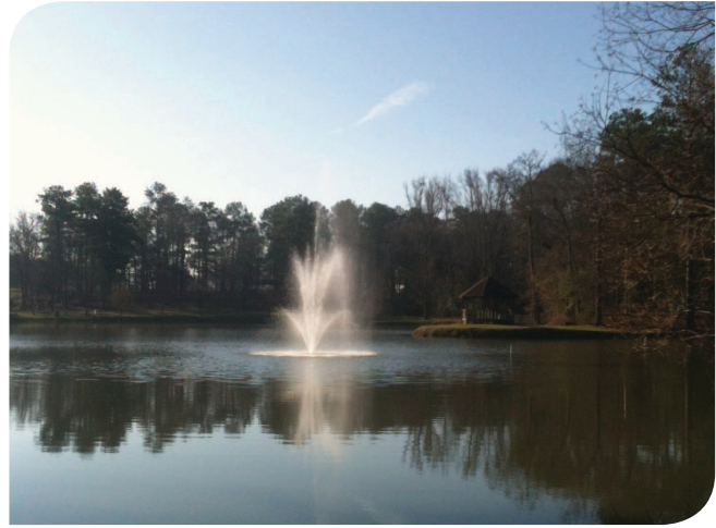
A hybrid geothermal system utilizes a local lake as its renewable energy source and heat sink.
