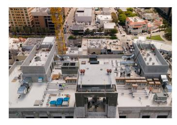
The system design addressed the building's unique acoustic requirements by strategically placing VRF outdoor units across the roof, 6th floor, and 3rd floor. This configuration, enabled by VRF's flexible piping design, minimized noise impact on the penthouse while maintaining improved performance across all 20 floors.
