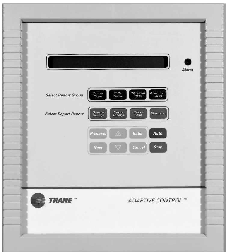
Figure 8 - Unit control module with Clear Language Display Keypad (UCM-CLD)
