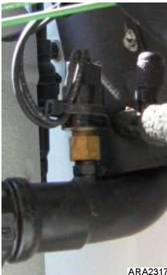
Low Pressure Cutout Switch Installed
