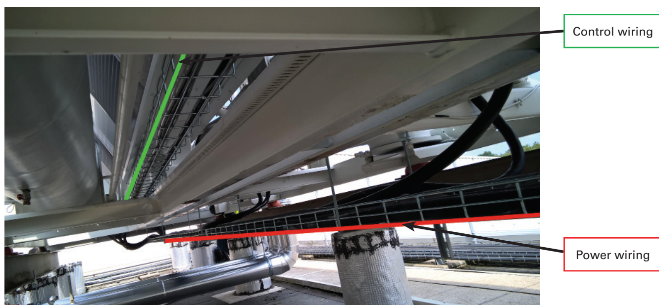
Figure 12 - Wiring installation
