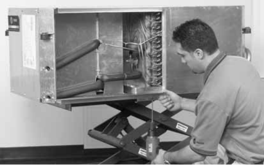
Figure 52. Install top/bottom filter rack
