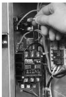
Figure 64. Connecting speed-tap wire
