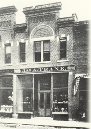
Trane Storefront La Crosse, Wisconsin 1891
