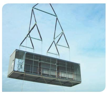
Many Trane custom units are shipped completely assembled, ready to rig into position with one single-point power connection.
