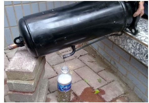
Figure 6-2.8: Draining oil from a compressor
