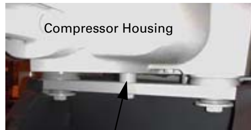
Figure 8. Compressor shipping spacers B family (discharge side)
