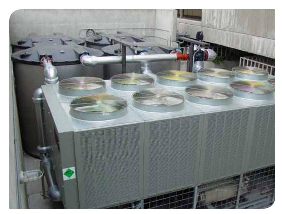
One way Trane reduces energy costs is with a thermal storage system design that uses ice made at night, when energy demand and cost are lowest, to cool the building during the day.
