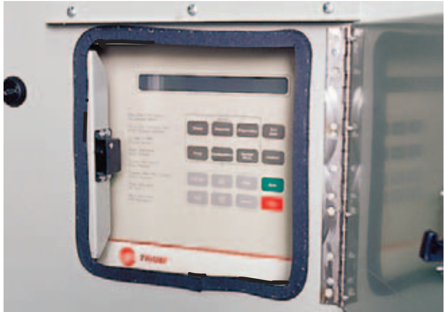
Figure O-GI-1. The human interface panel on the Trane Packaged Fresh Air unit
