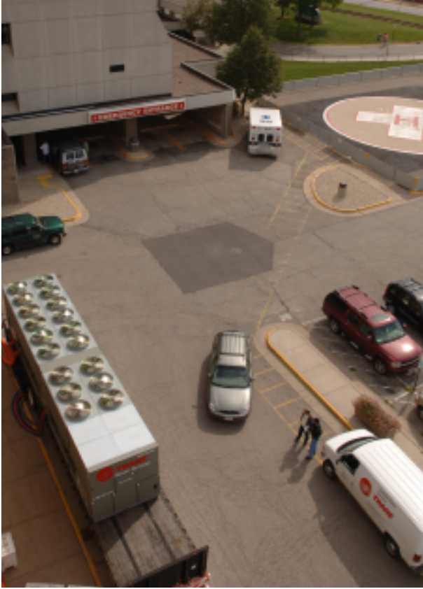
Overhead shot of a temporary unit.
