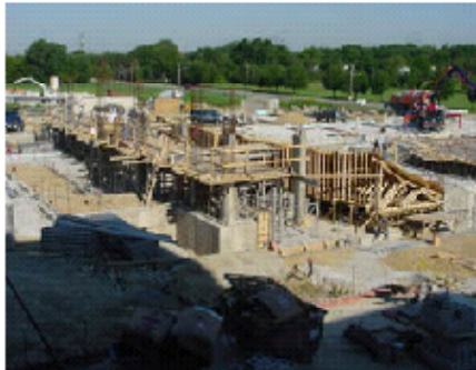
Bolingbrook High School under construction
