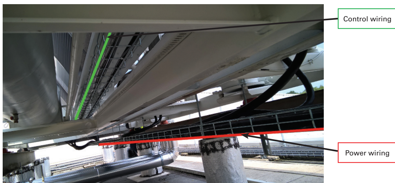
Figure 12 - Wiring installation
