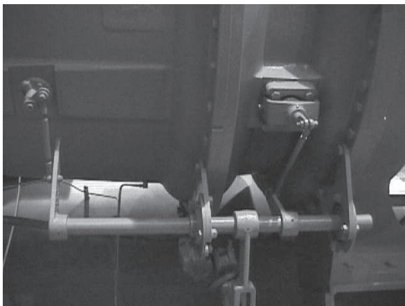
Figure 12. Vane actuator operator mechanism
