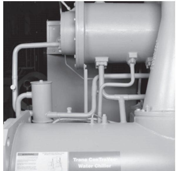
Figure 14. Lubrication system motor cooling lines
