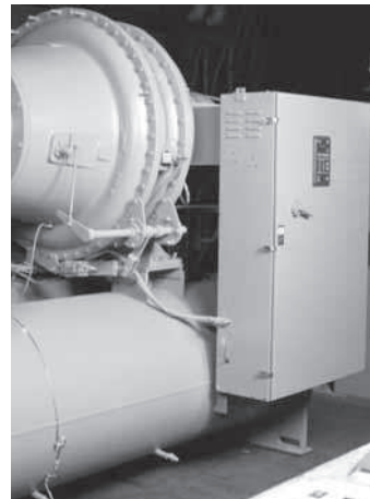
Figure 20. Starter mounting bracket
