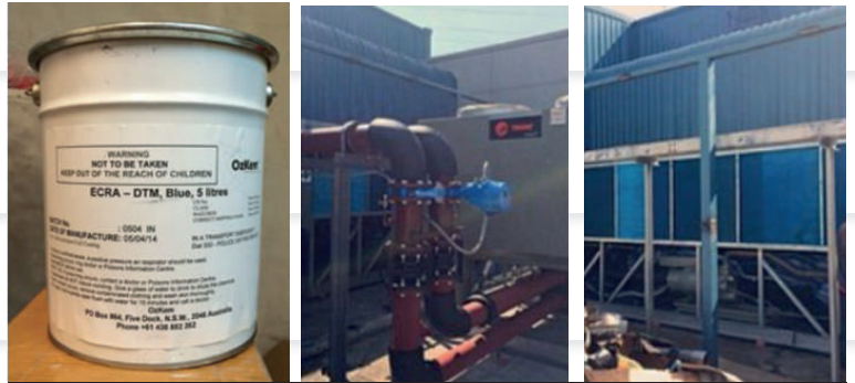
Anti-corrosion TR-DTM (On-site Coating Spray)
